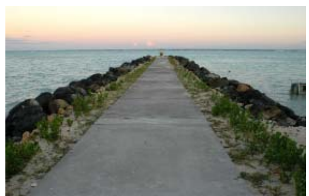
Groin structure assists in beach stabilization and becomes an attraction for tourists.
