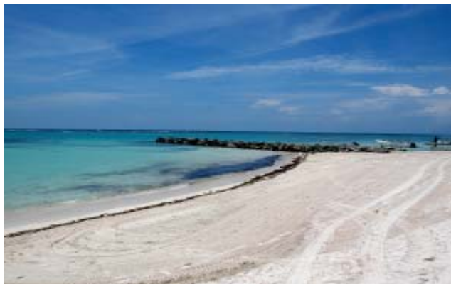
Groin structure and interventions have added approximately 33 feet (10 meters) in coastal and submerged sand area.
