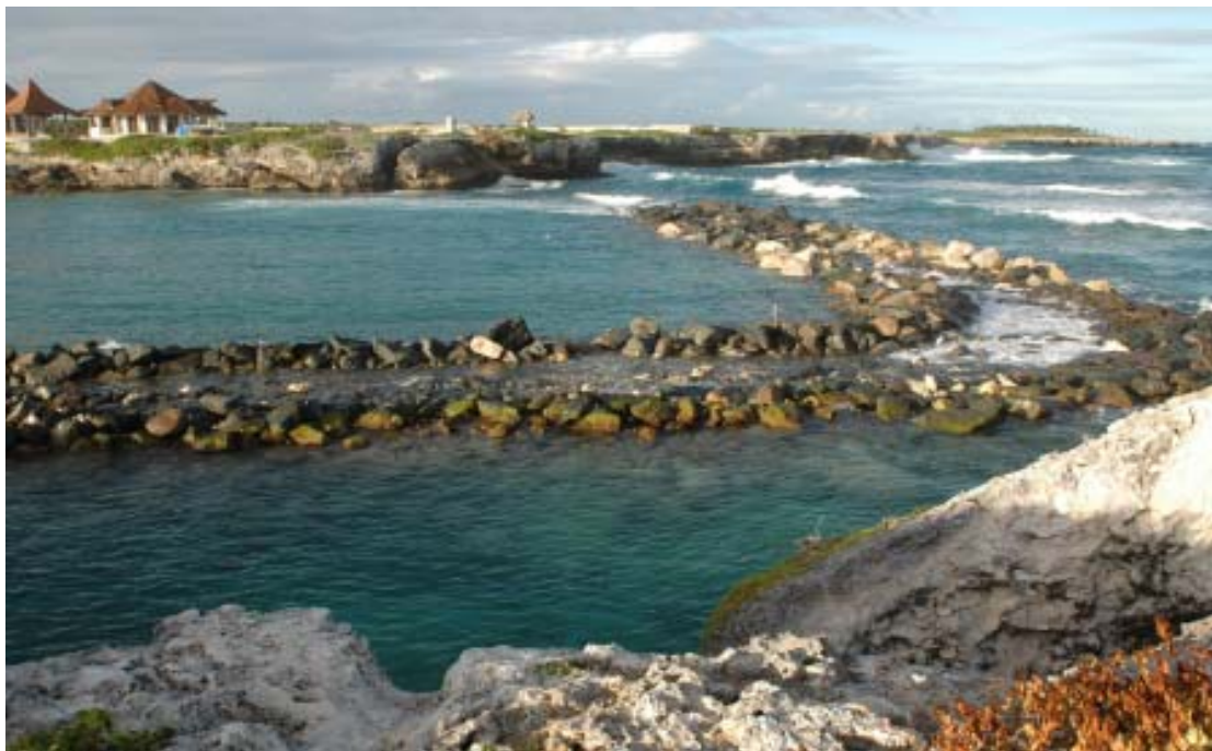
Corales Cove breakwater initiated in November 2005.
