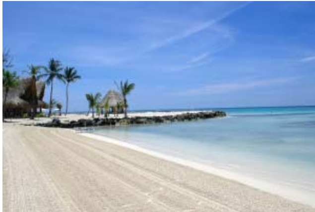
The circular groin has been instrumental in stabilizing the beach and accumulating sand in the south beach of PUNTACANA Resort & Club.
