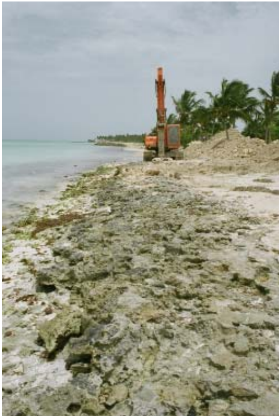
Exposed rock was cut to create catchments for sand nourishment.
