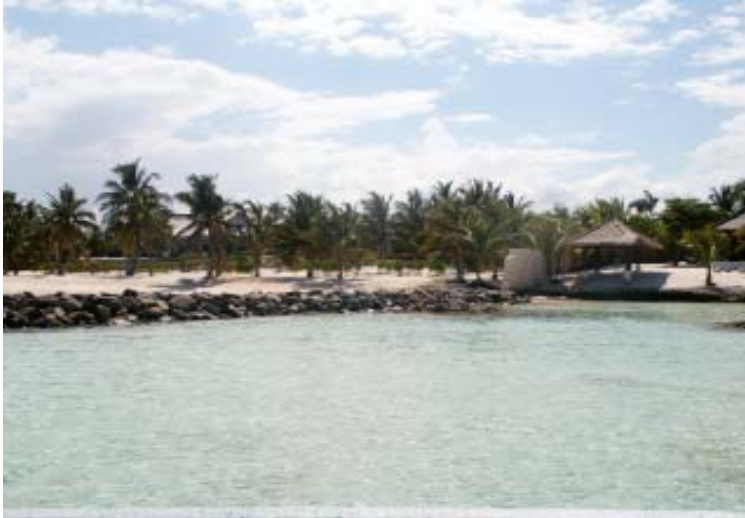
A groin structure was built between Corales #3 & #4.
