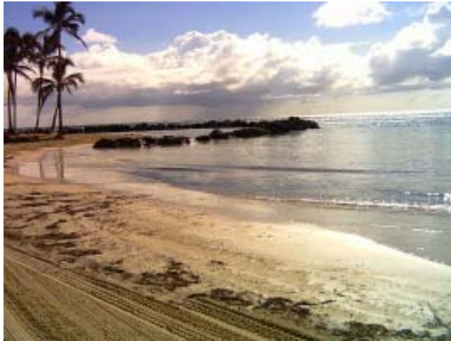
A circular groin structure was built to imitate the original coastline that had eroded over the last decade.
